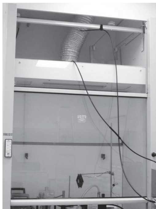
Figure 13: Required accesses to the exhaust duct
