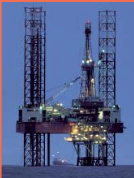
Olieplatform Hoa Qui/FN
